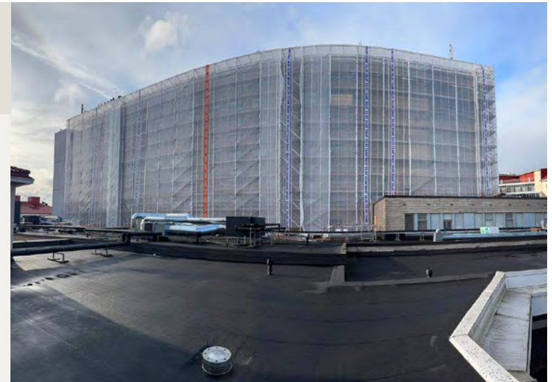
The facade renovation of Tyks Mäntymäki Hospital began in September 2025.
